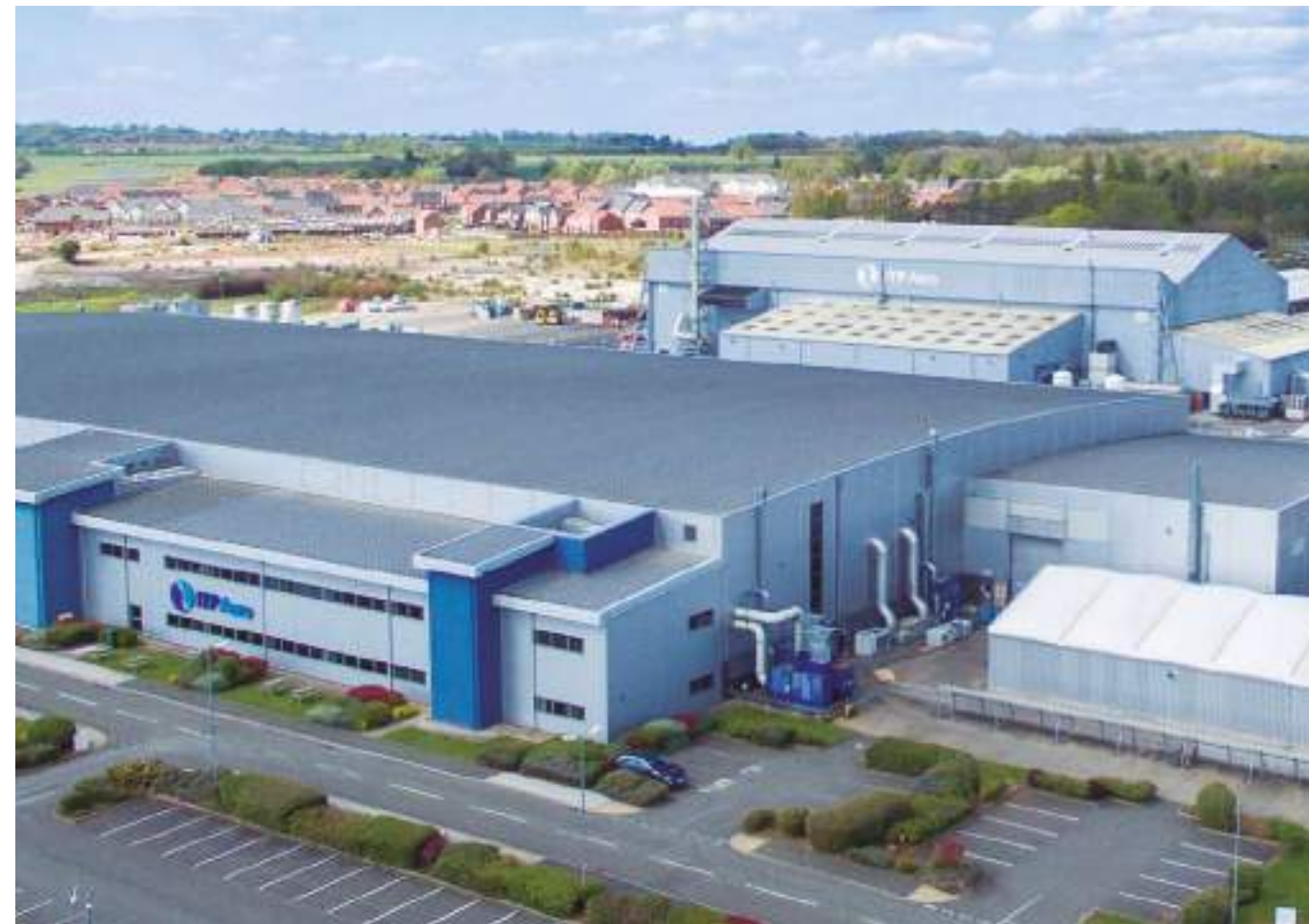
ITP Aero facilities in Hucknall (United Kingdom).
